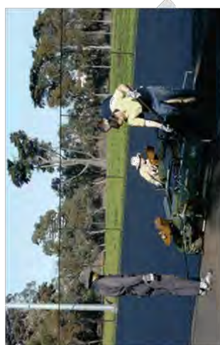
Photo 32: In-situ Shockpad being laid (Source: Pajanti)
