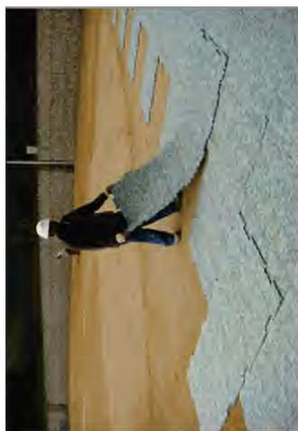
Photo 31: Prefabricated Shockpad being laid (Source: TEAM Sports)
